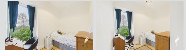
Single glazed window and double radiator.
